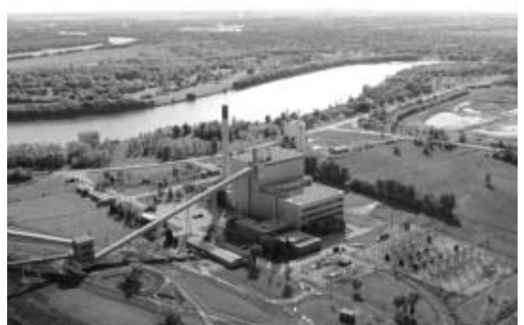
Originally built in 1960, the 121-megawatt (MW) Selkirk Generating Station plays an important role in Manitoba Hydro's electricity system as a backup to the utility's hydroelectric sources.
