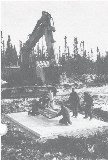
Insulation in place to prevent thawing causing the tower to settle.
