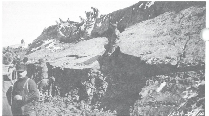
Sliding displaced material into the east trench.
