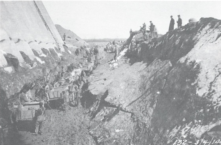
The east trench showing excavation by horse and cart.
