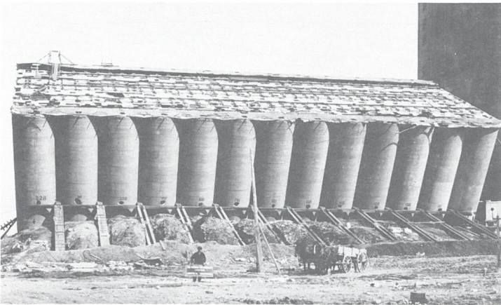
The west face of the elevator with the "pushers" installed.
