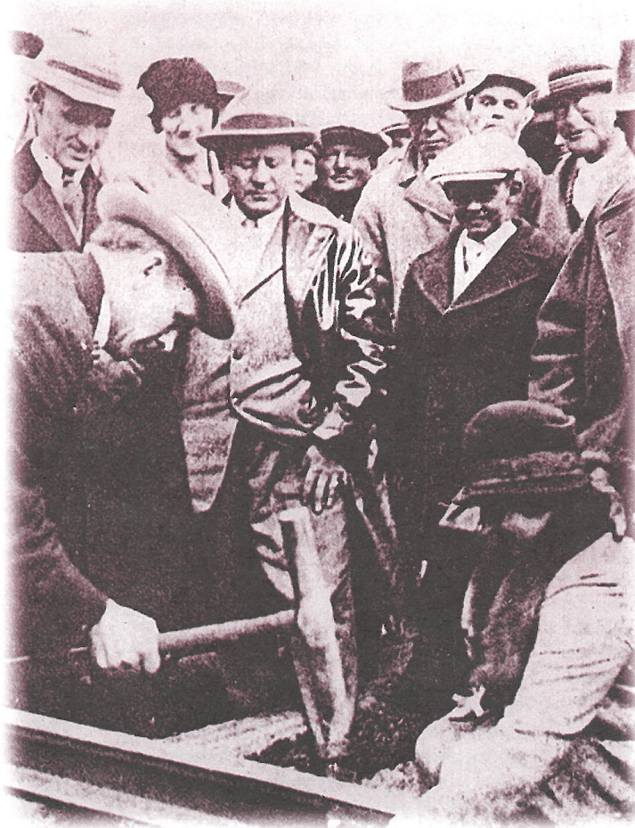
Mrs. McLean and the Hon. John Bracken of Manitoba drive the last spike on the Manitoba Northern Railway of the CNR.
