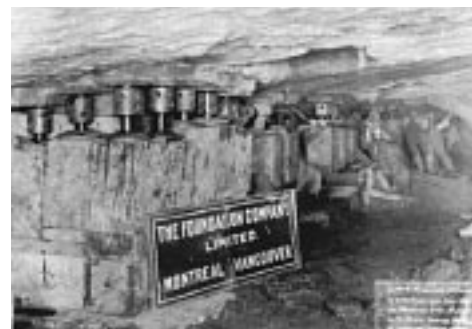
Shoring screws used to lift 20,000 ton binhouse.
