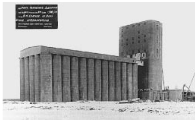
Transcona Grain Elevator after straightening.
