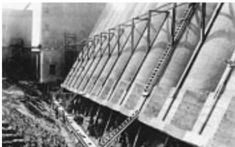
Excavation on East side of bins.
