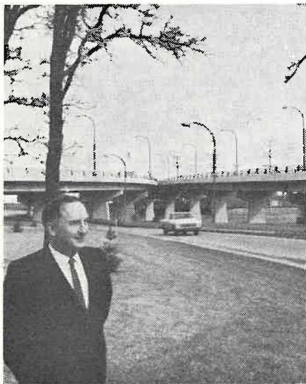
C. H. Templeton, P. Eng., shown at the St. James Bridge and Interchange.
