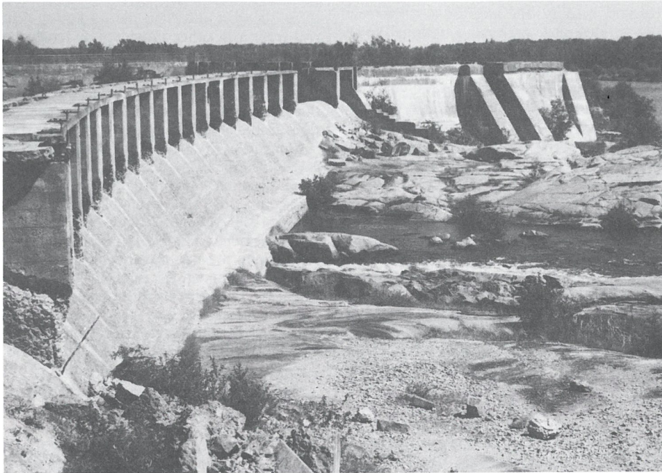
Spillway and Forebay.
