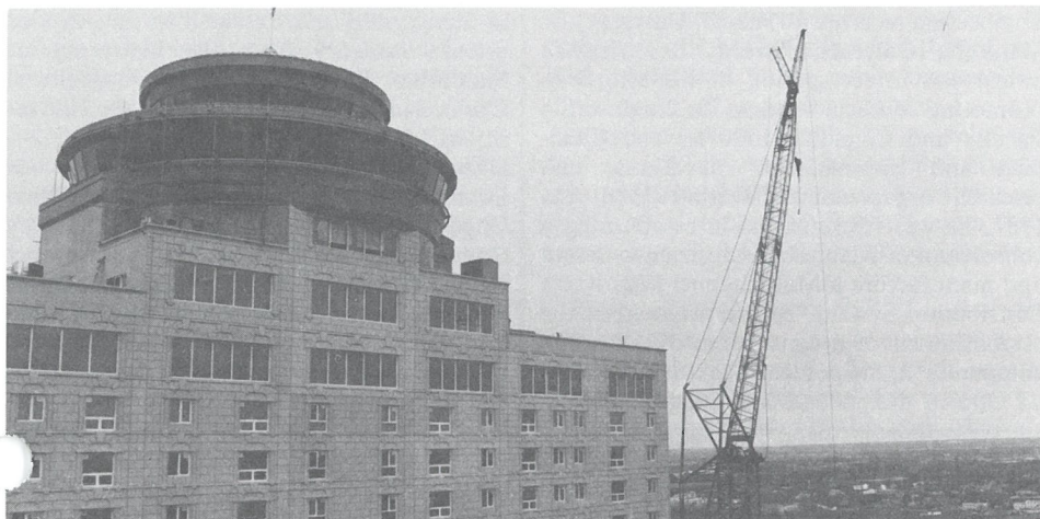
Revolving Restaurant, 200 Ton Crawler Crane.
