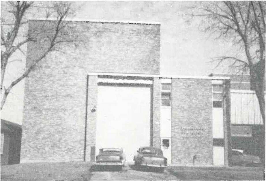
FETHERSTONHAUGH HIGH VOLTAGE LAB (See story inside — Canadian Standards Association)
