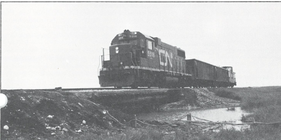
Test train at bridge site near Grosse Isle, Manitoba.
